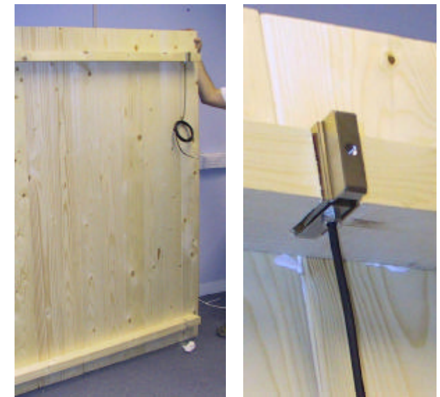
Fig. 4. The floor when it was installed in upright position (left). Enlarged view of the load cell embedded into the floor (right).
